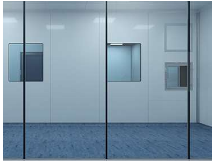
Cleanroom panel work
